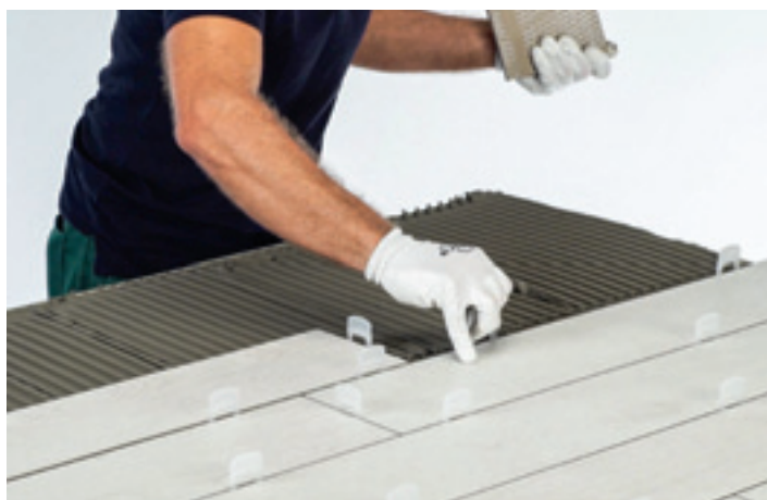
disposable clips installation
