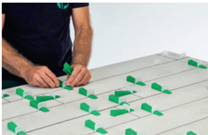
levelling wedges insertion
